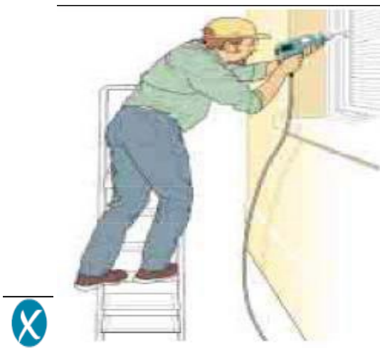
Incorrect – steps side on to work activity
