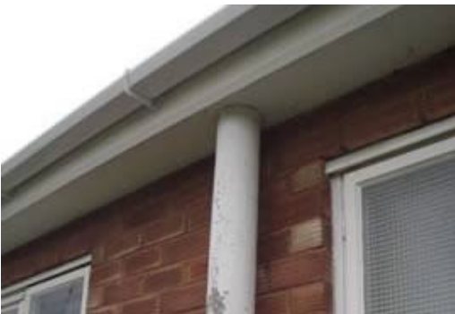
Asbestos cement drainage pipe (downpipe)
