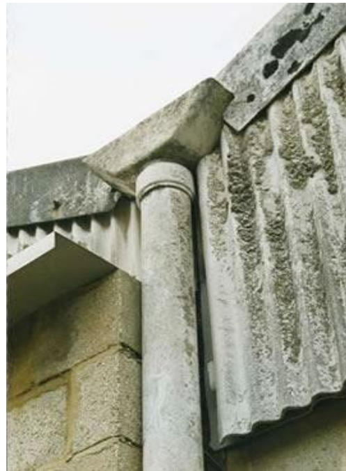
Asbestos cement downpipe, hopper and profile sheet
